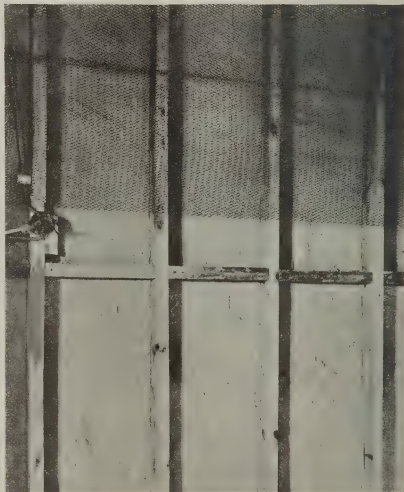
BACK PLASTER APPLIED
